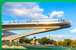
Floating Bridge Moscow
